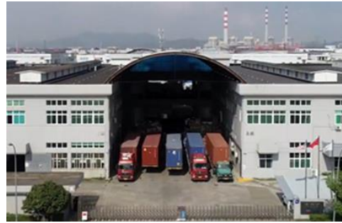
Ningbo Facility – integrated distribution
