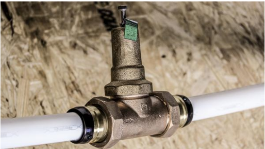
Pressure regulating valves
